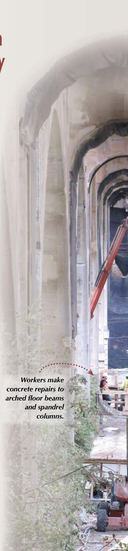
**Workers make concrete repairs to arched floor beams and spandrel columns.**
