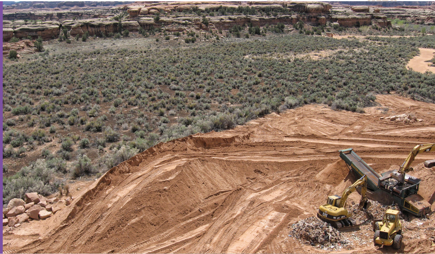
The soil-waste separation technique used at Canyonlands saved "golden soil," enabling Michael Baker to restore the site more economically.
