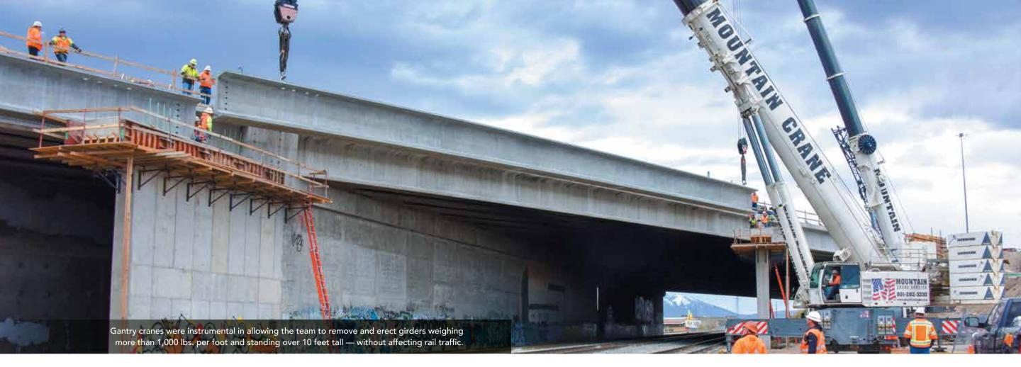
Instead, the team devised an ingenious solution — build giant gantry cranes on site to facilitate bridge widening and narrowing, then disassemble the cranes and remove them once the work was completed. The gantry cranes were instrumental in allowing the team to remove and erect girders weighing more than 1,000 lbs. per foot and standing over 10 feet tall — without affecting rail traffic. It was a remarkable feat, a sight that caused even veteran engineers to marvel.
