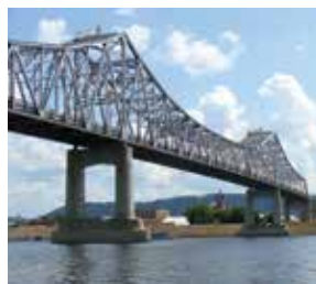
Winona Bridge Rehabilitation and Reconstruction Project (Grand Award)
