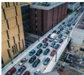
Courtland Street Bridge Replacement (State Award)
