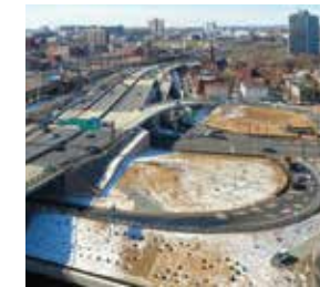
I-280/Route 21 Interchange Improvements Project (Platinum Award)
