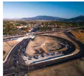
I-15/Temecula Parkway Interchange (Merit Awards)
